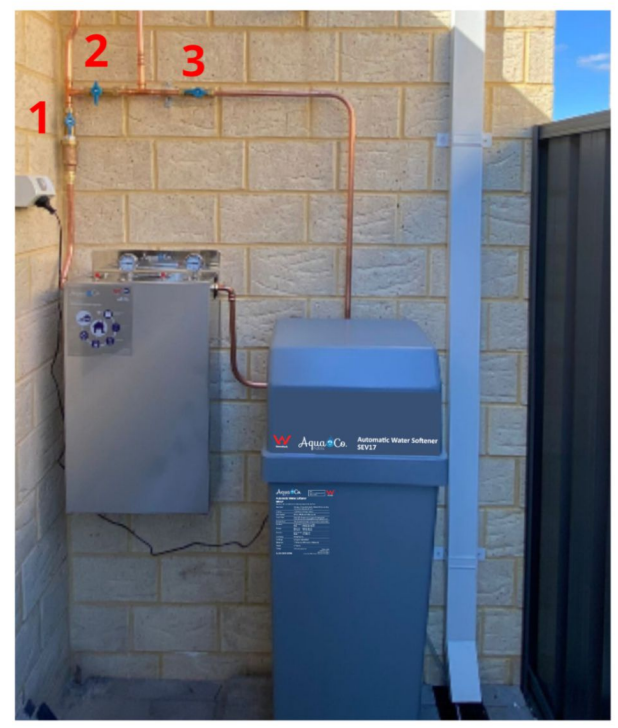
Valves 1 and 3 remain open. Valve 2 remain close.
