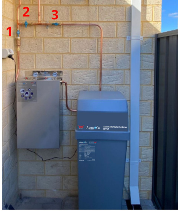
Valves 1 and 3 remain open. Valve 2 remain close.
